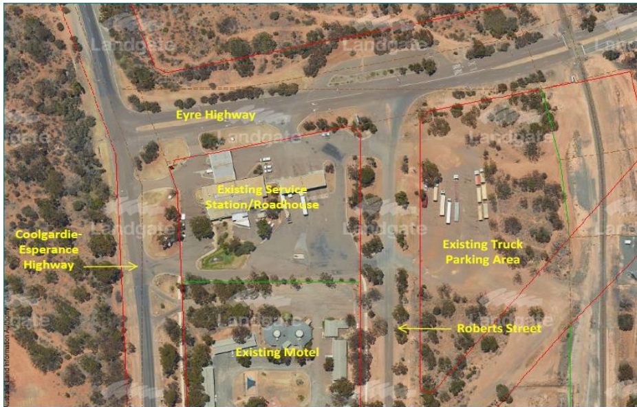
Figure 2 Aerial Image denoting the site context of lots 2 and 3
