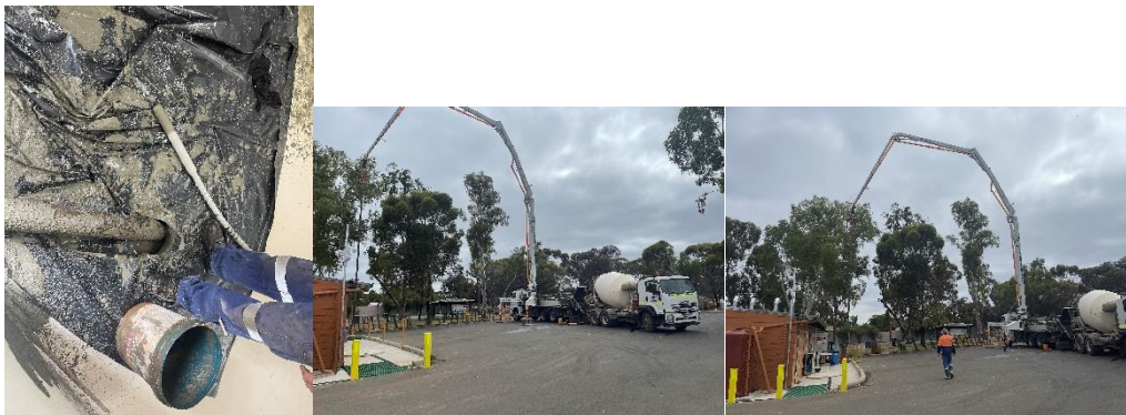
LAUNDRY FLOOR VOIDS BEING PUMPED FULL OF CONCRETE SLURRY
