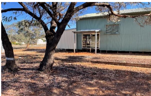
MENS SHED SLIDING DOOR IN PLACE.
