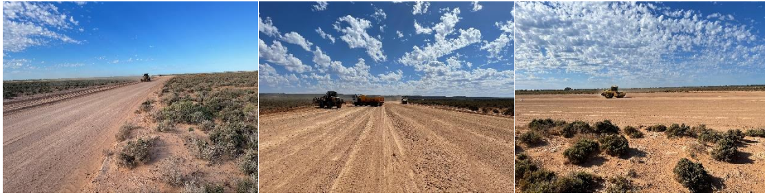
EUCLA ROAD AND AIRSTRIP WORKS
