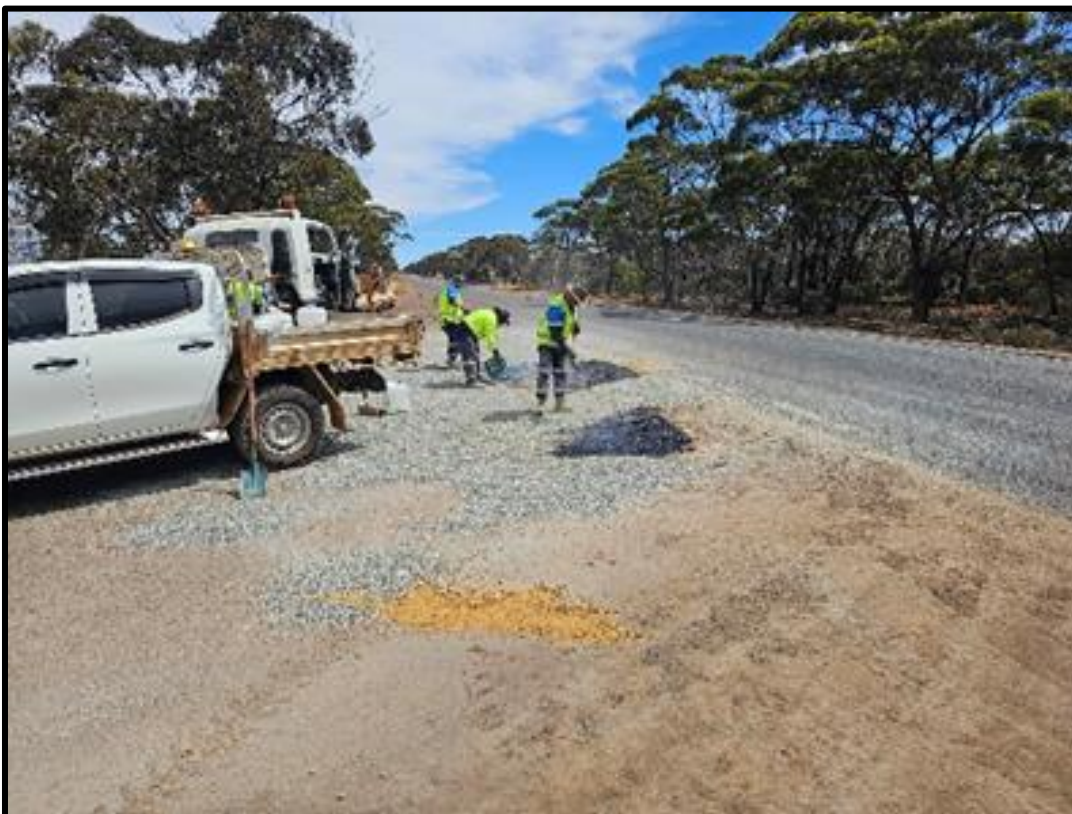
Private works at the OK road intersection
