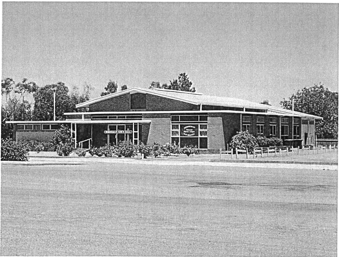
Shire of Dundas - TOWN HALL
