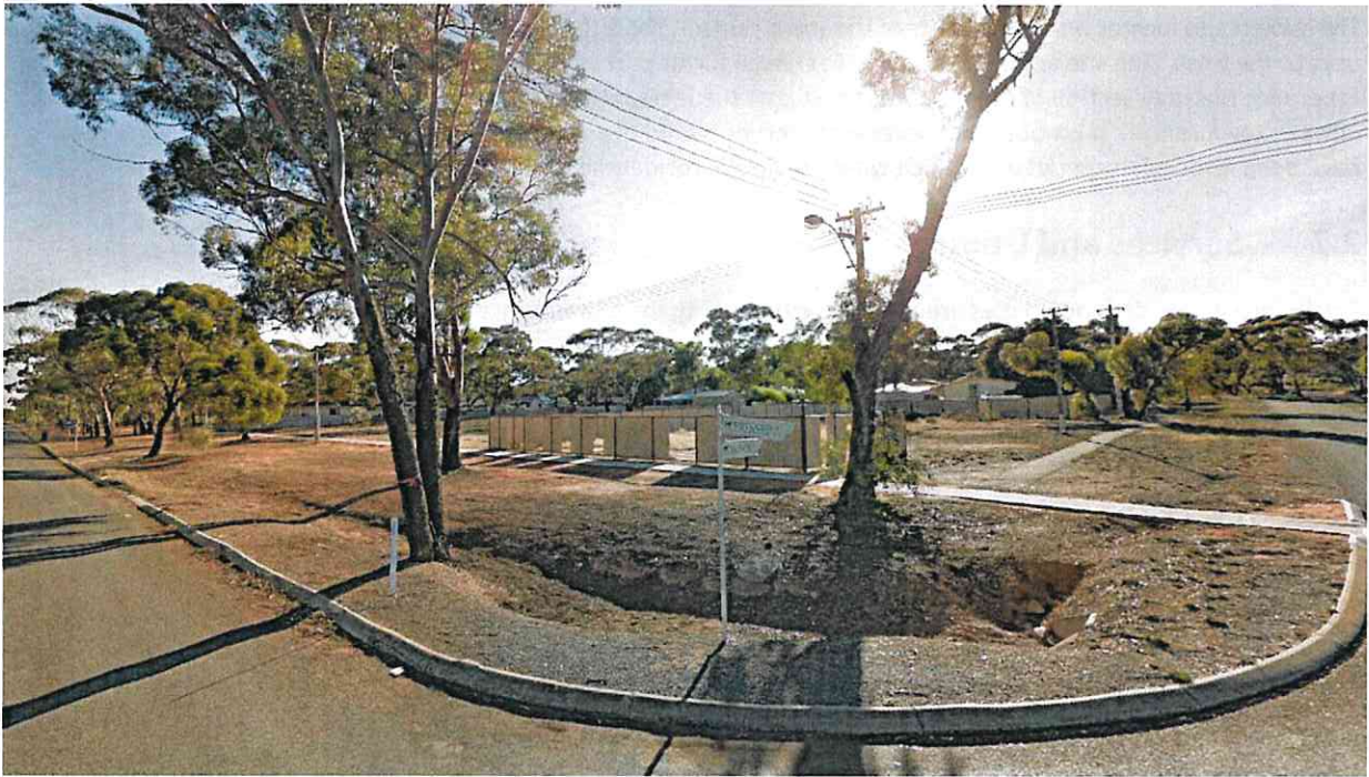
Figure 2: Site appearance from corner of Prinsep St and Mclvor St (Source: Google)
