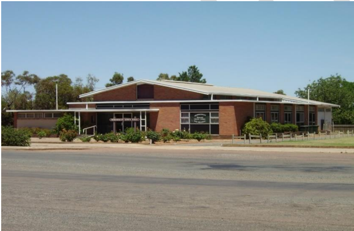
Shire of Dundas – Town Hall
