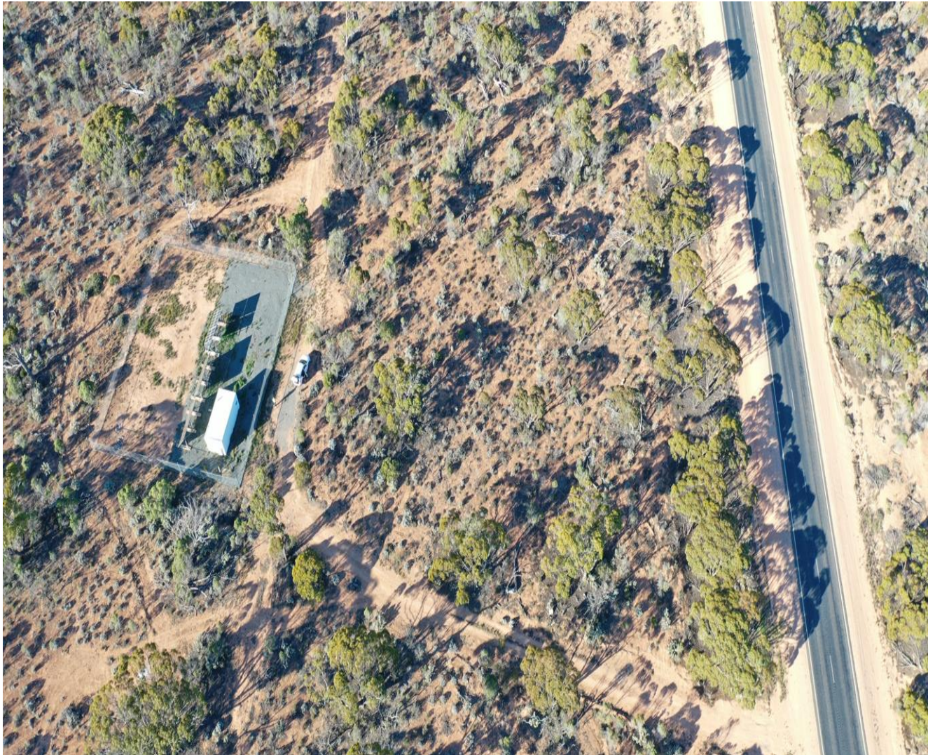
Aerial Image – Telstra ‘Virginia’ Telecommunications Facility
