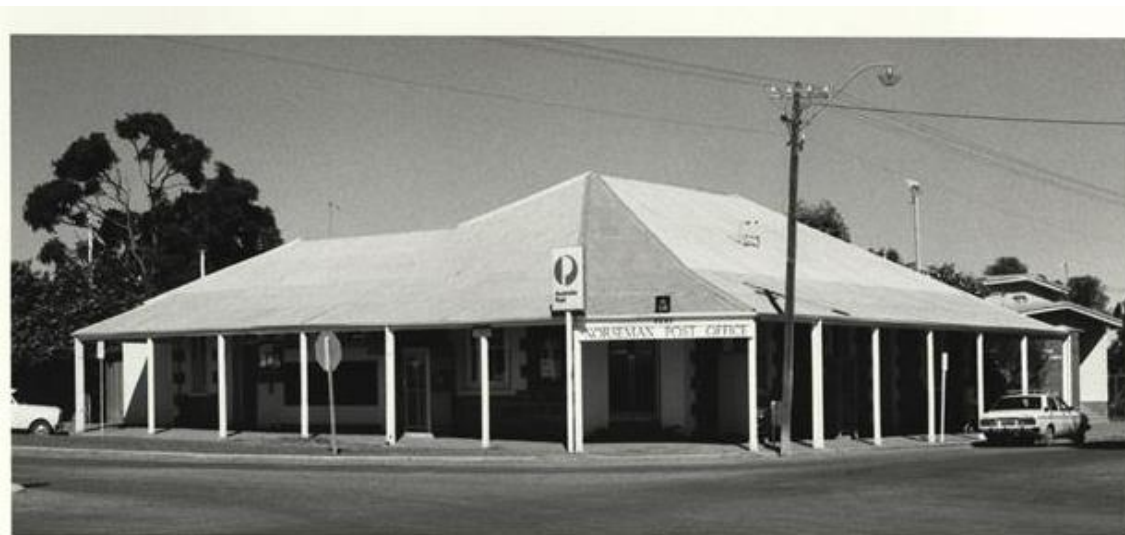
Figure 3 - 1983 Photograph of the former Norseman Post Office
