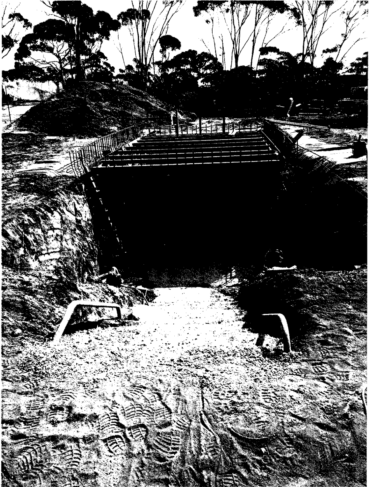
The above photo shows the magnitude of the formwork and re-enforcing steel that went into the project
