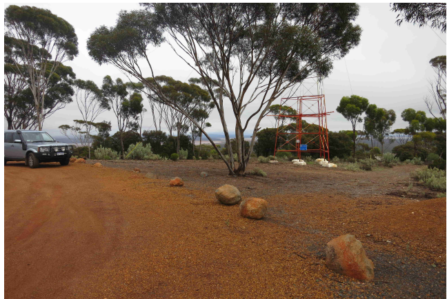
Inadequate rock bollarding is another issue to be addressed in the site upgrade (below)
