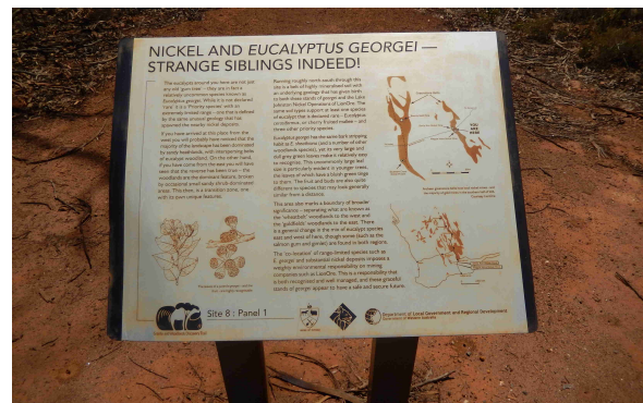
Panels left undeanned for too long eventually become stained, unattractive and hard to read. Note also damage to lower left corner
