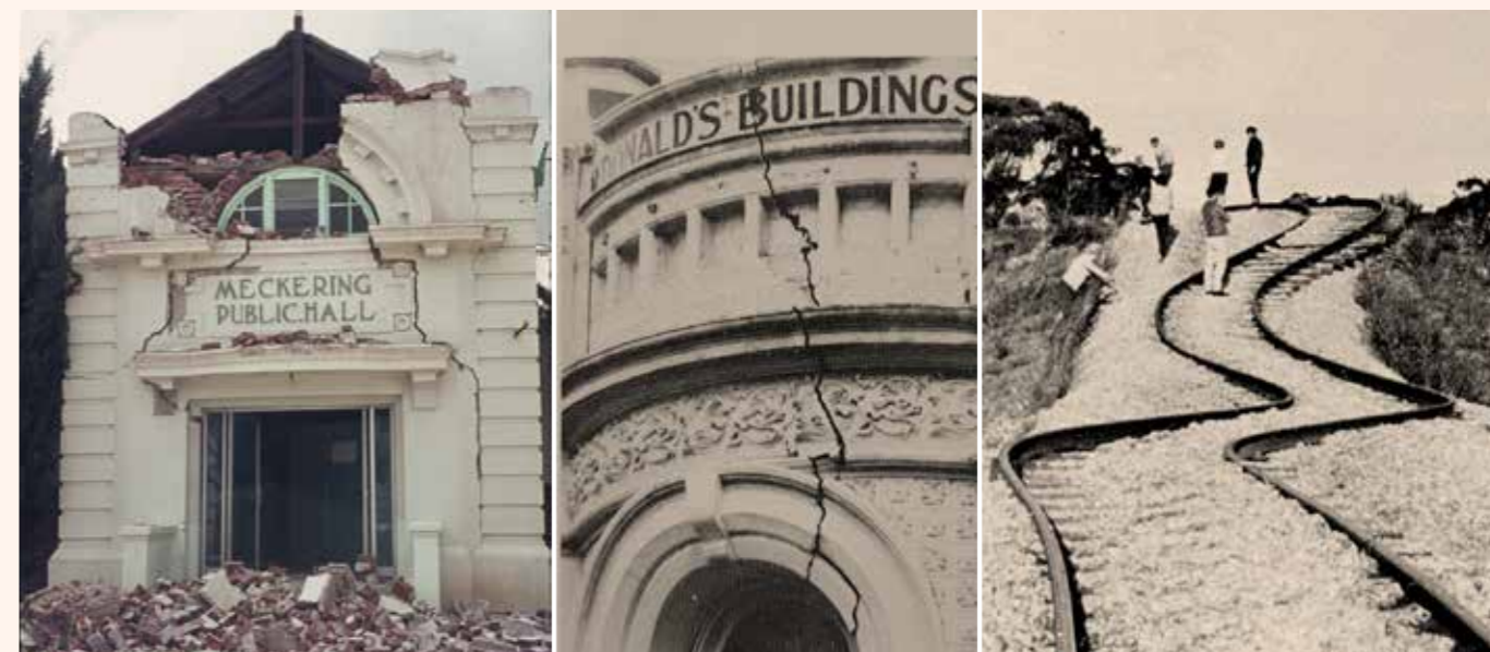
Figure 1: Damage resulting from the 1968 magnitude 6.5 Meckering earthquake. Damage to the Meckering Town Hall (photo to the left: State Library of Western Australia); McDonald Building at the corner of Barrack and Murray St, Perth CBD (photo at the centre: © WEST AUSTRALIAN NEWSPAPERS LIMITED); and rail lines bent due to deformation of the ground surface (photo to the right: Johnston and White, 2018).
