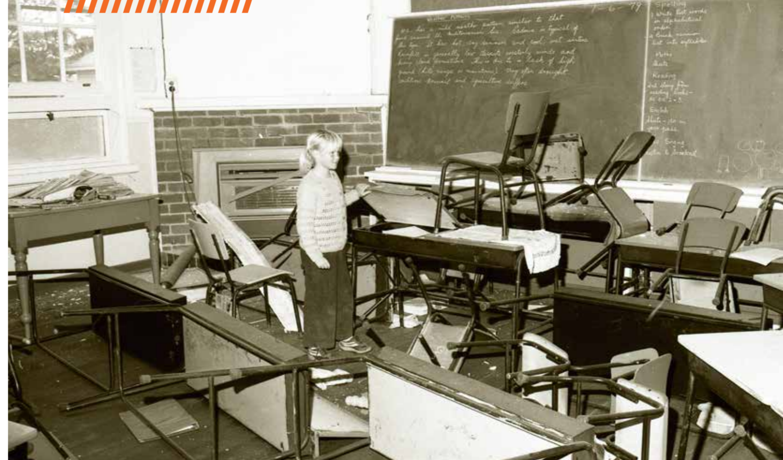
Damage in school during the Cadoux earthquake (1979) © WEST AUSTRALIAN NEWSPAPERS LIMITED.
