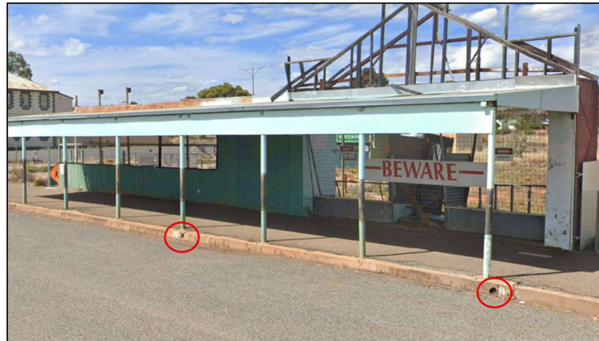
Figure 2: Existing Stormwater Discharge Pipes
