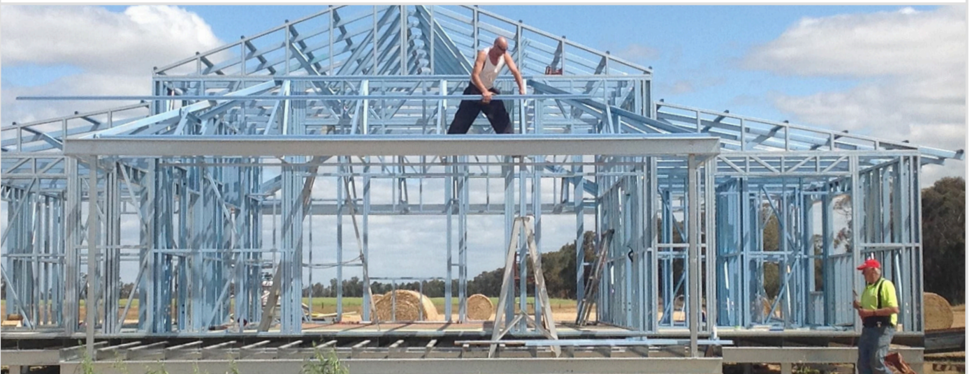
Customer-managed build in progress on a stud frame kit.
