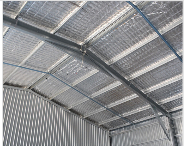
Internal view of a portal framing system pre customer-managed fit out.
