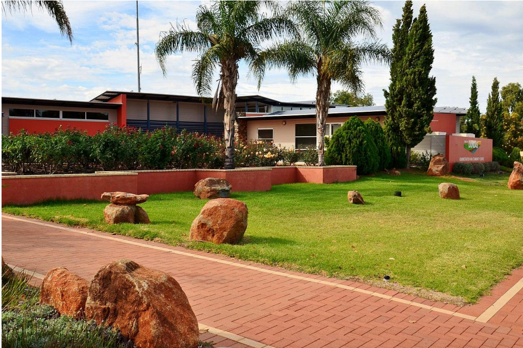
Shire of Dundas Administrative Offices, Norseman
